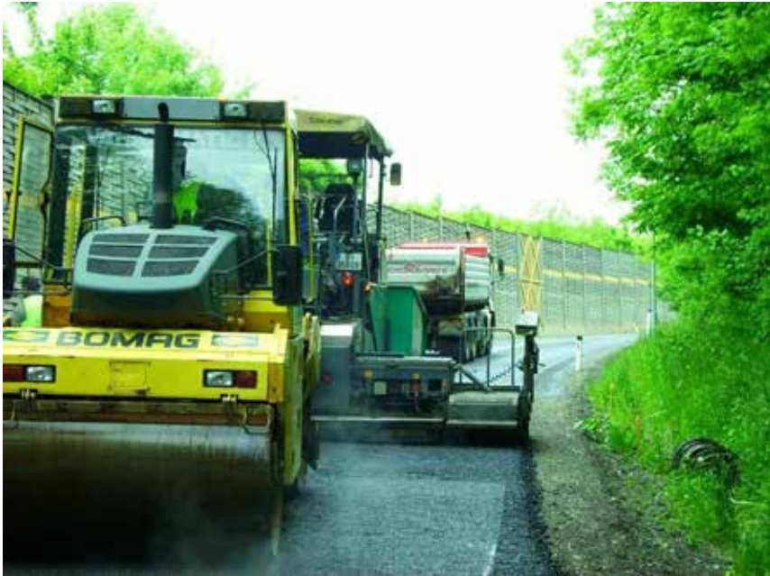
Paving of AC trag
