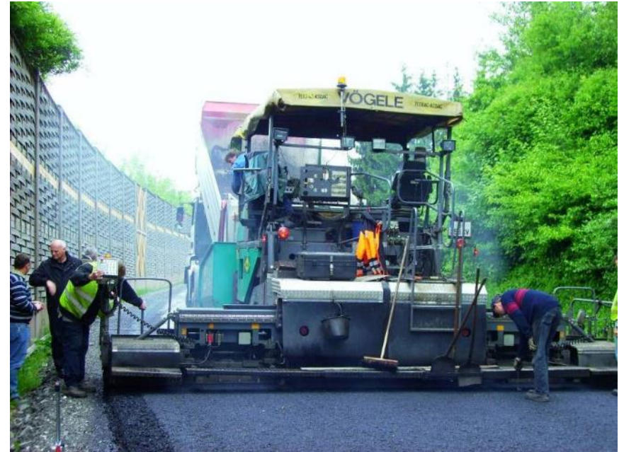
Paving of AC trag
